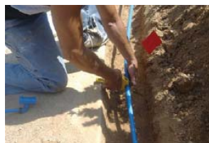
2. Cut-into the lateral line
