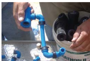
1. Assemble Blu-Lock swing joints on-site
